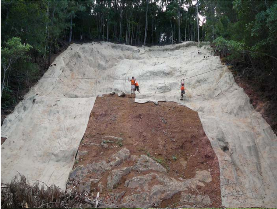
Jute matting installation for QR on a slip near Barron Falls:
